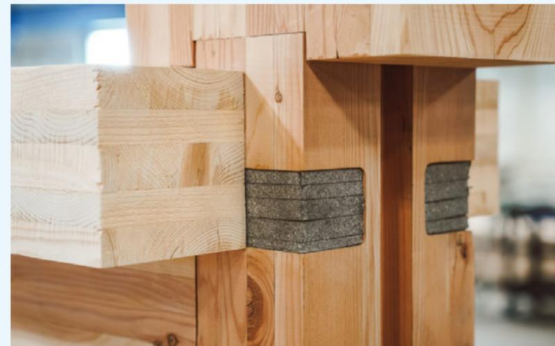
assemblies and wet-applied materials are significant barriers to deconstruction as it becomes difficult, costly, and potentially impossible to isolate and remove those products from one another for reclamation, usually making the entire assemblies landfill waste. To reduce these types of challenges, in addition to the mortise and tenon joints, Timberlab added cuts by CNC machines to install intumescent fire tape instead of traditional wet-applied
